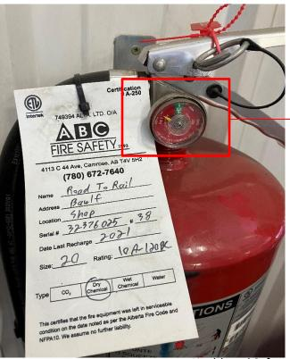
This fire extinguisher is *Undercharged*, as shown on the pressure gauge. If this extinguisher was used to fight a fire, the required pressure may not be enough to be effective.
