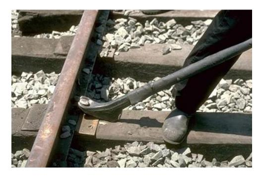
Example of a claw bar being used to remove a spike
