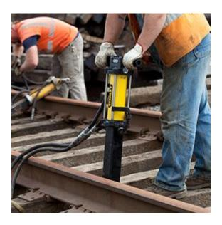
Example of a hydraulic spike puller being used to remove spikes
